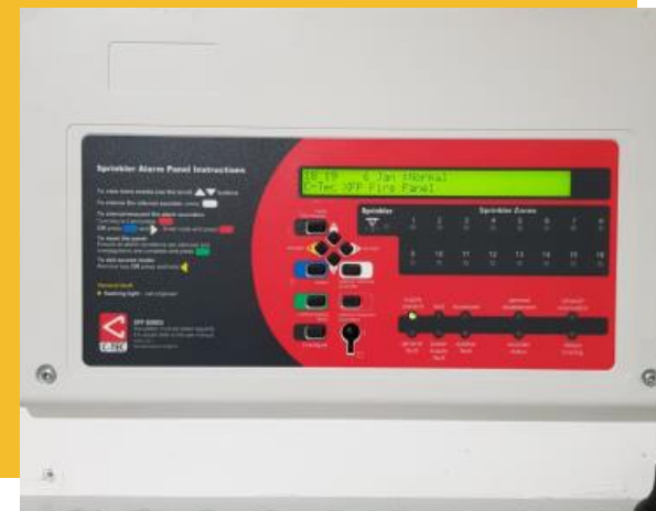
Sprinkler Alarm Panel
